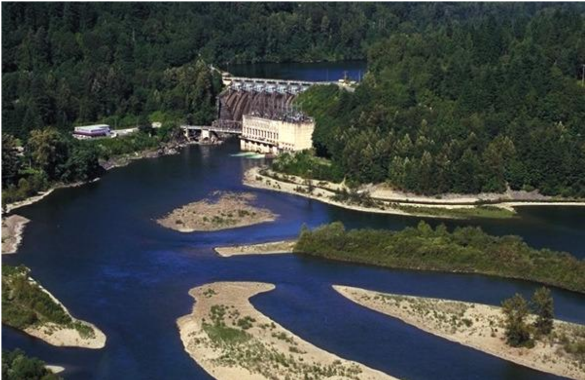
The Ruskin dam came online in 1930, and it now requires rebuilding at a cost of about $800 million.
